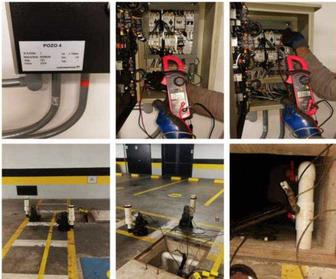
**FIGURA 8 POZO 4 EQUIPO NIVEL FREATICO**
